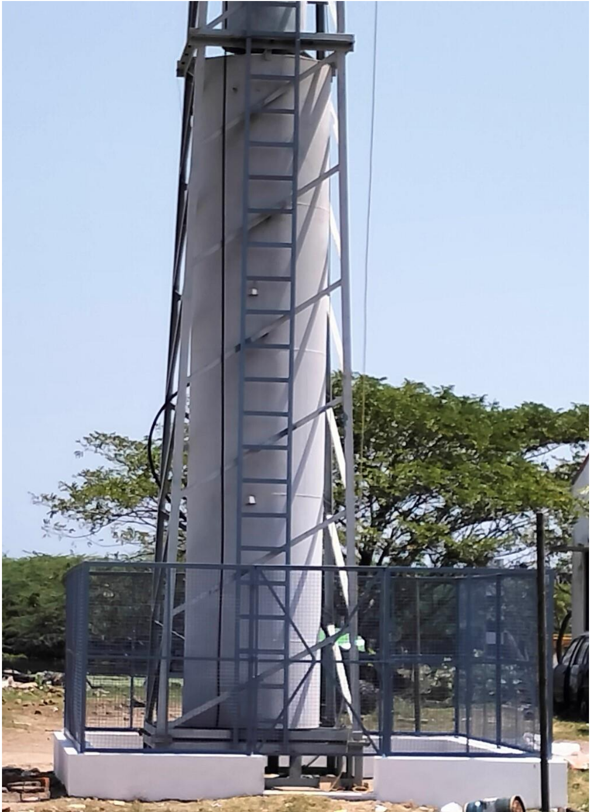
Fig 3: Ladder and Fencing
