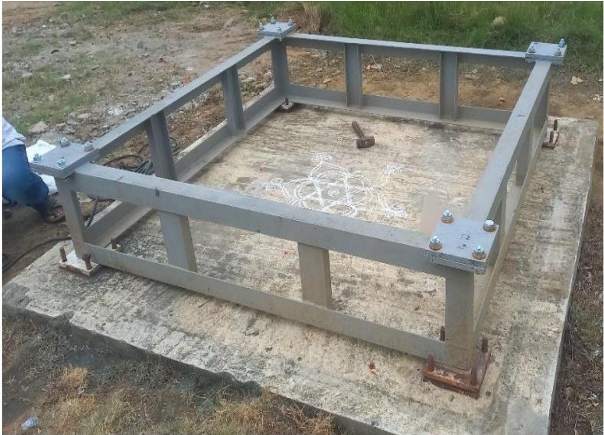
Fig 2 : Tower Foot Extension structure fixed over the foundation.
