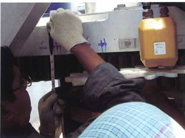
Nacelle Instrumentation work for Inox 2000 kW Wind Turbine
