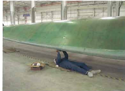
Blade Instrumentation work carried out for WinWinD Power Energy for 1 MW Wind Turbine at Vengal, Chennai
