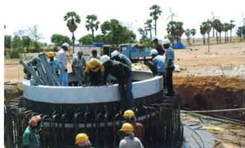
Foundation work is being inspected by UC, R&D and UC, WTTS
