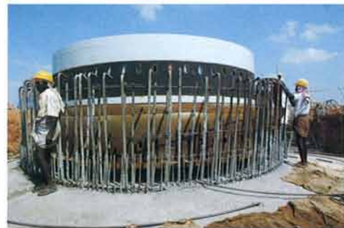
Foundation Work is in Progress
