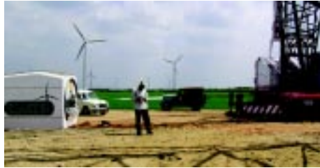
Provisional Type Testing of Pawan Shakthi (600 kW) Site survey at Senjuvadi
