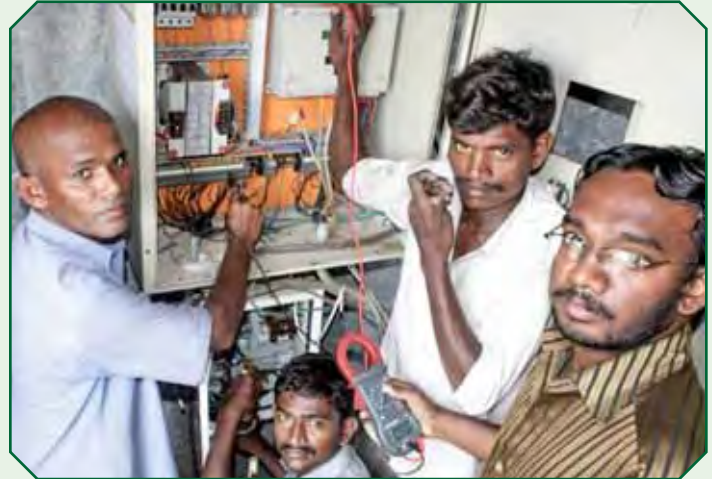
Maintenance of Panels of 200 kW Micon Machine
