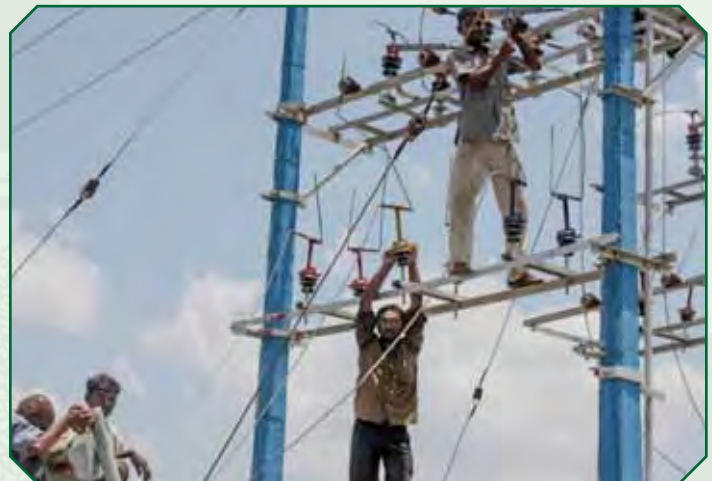
Preparation of 200 kW Micon Machine Transformer
