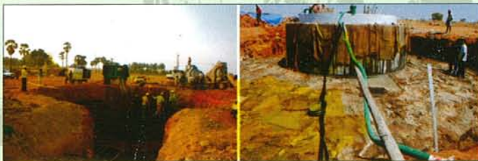
Foundation of the 2 MW R&D / Experimental Wind Turbine
