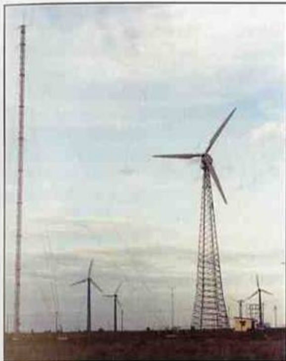
View of the Wind Turbine Test Station at Kayathar showing the Wind Turbine under test, Control Room and Wind Monitoring Mast
