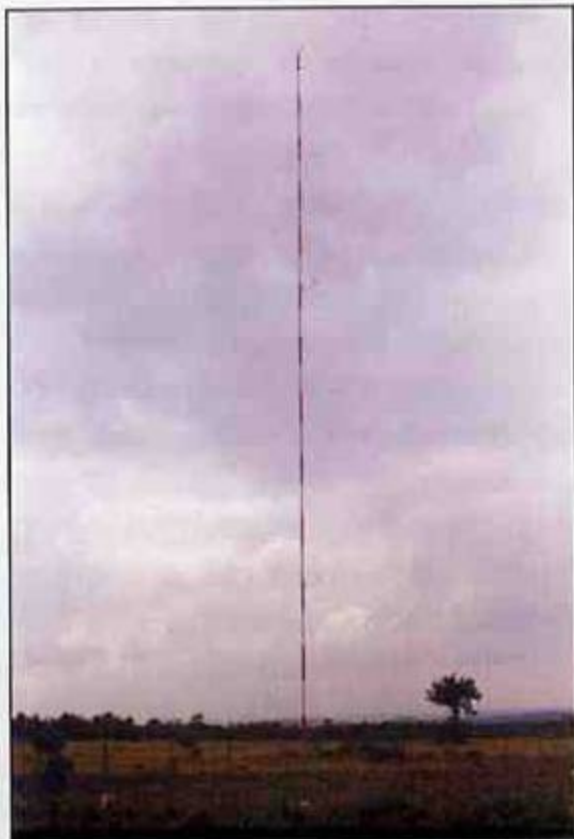
The 50m wind monitoring mast installed at Nelganti, Karnataka.
