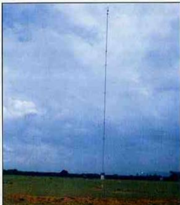
The 25m wind monitoring mast at Mylapatti, Tamil Nadu showing the sensors and data logger.
