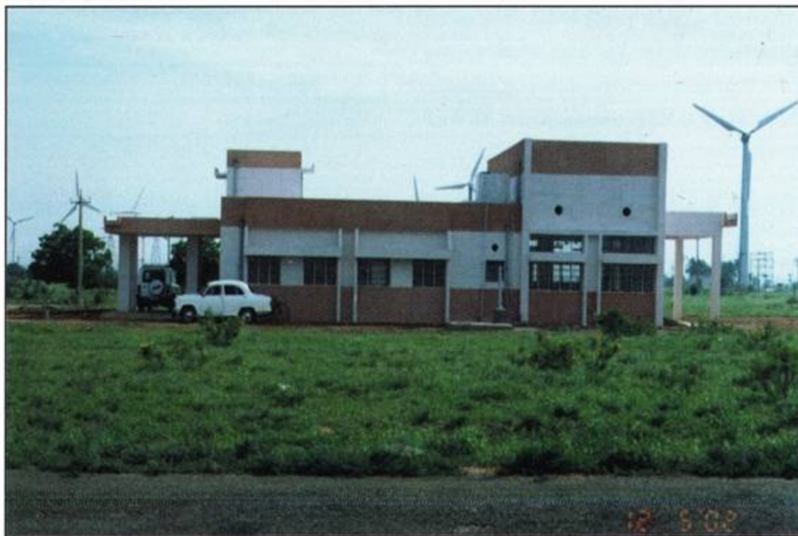
New building of WTTS
