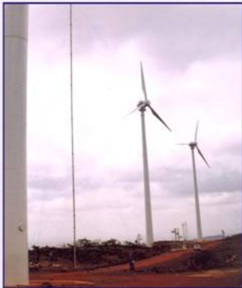
Power performance measurement on 230 kW Enercon wind turbine at Kapatguddah Hills.
