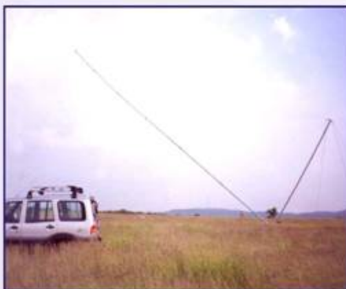
50m tall Wind Monitoring Mast being installed at Mahalunge, Konkan, Maharashtra.
