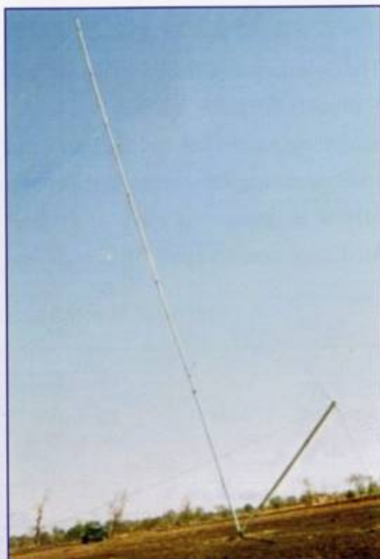
50m mast under installation at Dudha, Maharashtra
