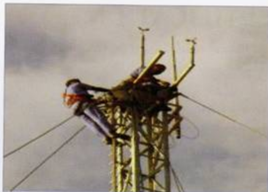
Instrumentation work on the mast for Provisional Type Testing on Enercon E 48 600 kW at Coimbatore
