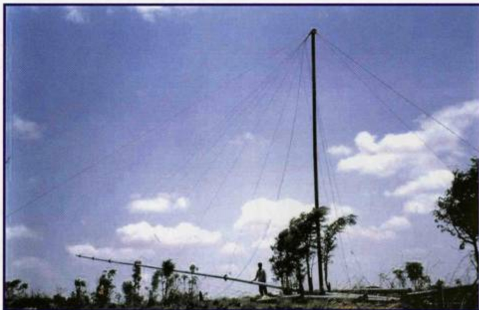
50 m tall instrumented mast under installation at T. B. Dam, Karnataka
