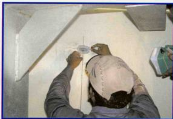
Engineer Strain gaging in turbine tower
