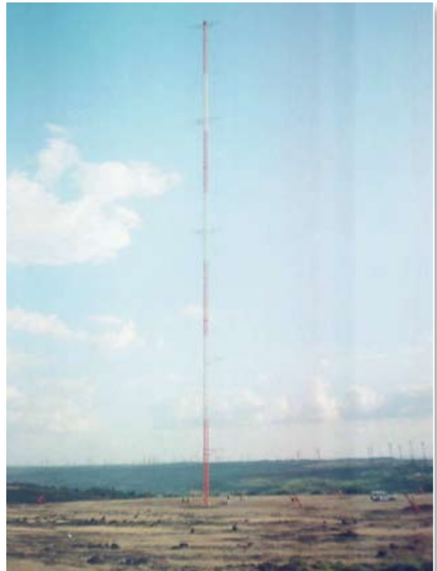
120 m mast installed at Jagmin, Maharashtra
