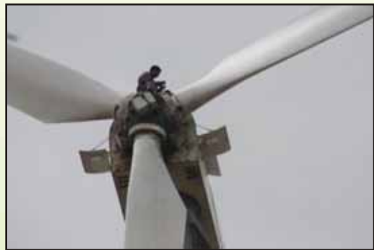
Wind Turbine Instrumentation at Site
