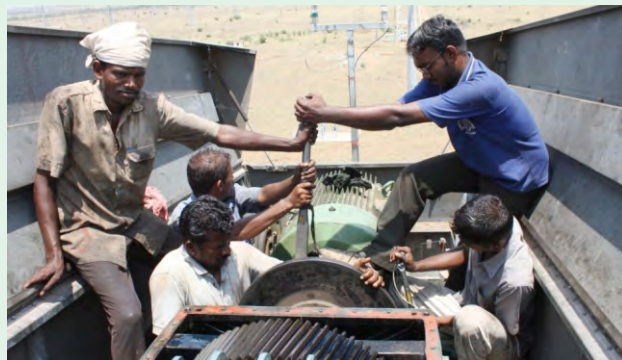
O&M of R&D wind farm at WTRS, Kayathar - Fixing of Generator Bearing
