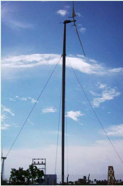
Test Turbine at Kethanur field measurements
