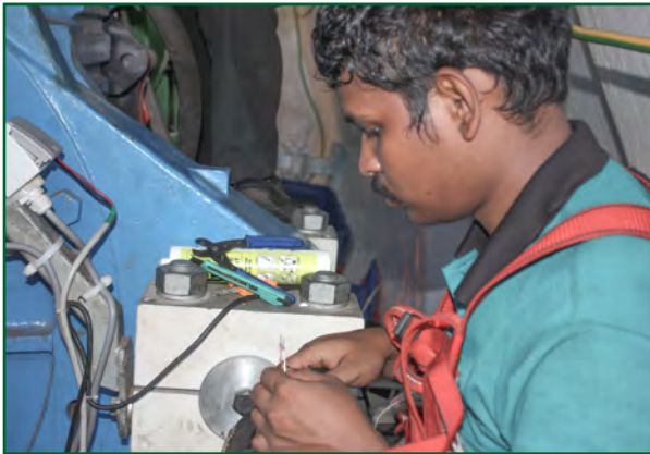
Yaw transducer wiring
