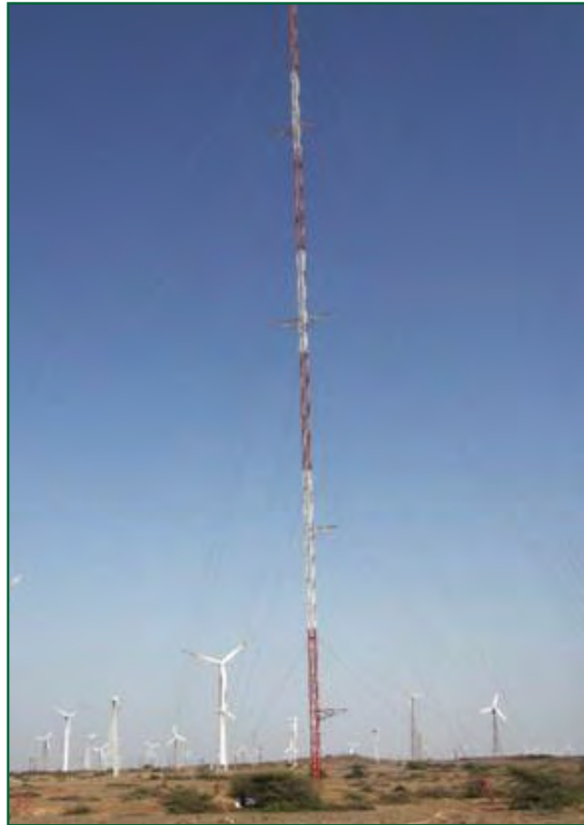
120 m tall lattice tower for wind measurement
