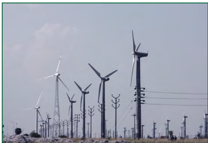
200 kW Micon Wind Electric Generators at WTRS, Kayathar
