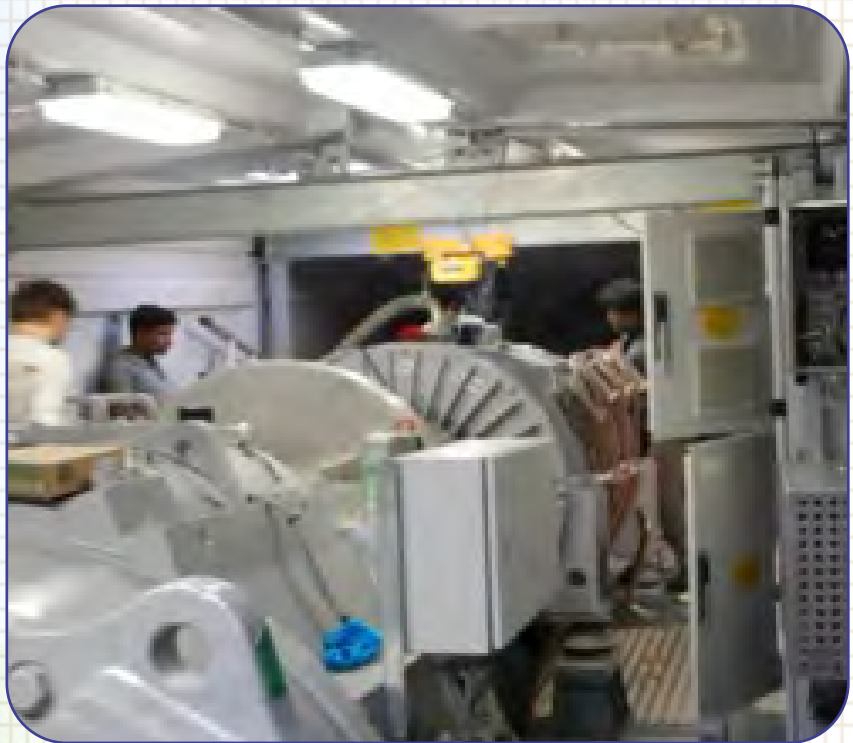
Condition Monitoring on the drive train
