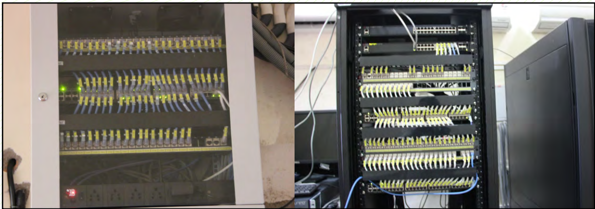
LAN Re-Structuring Work
