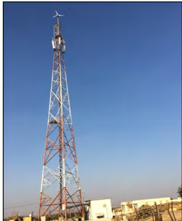
SWT installed on Telecom tower
