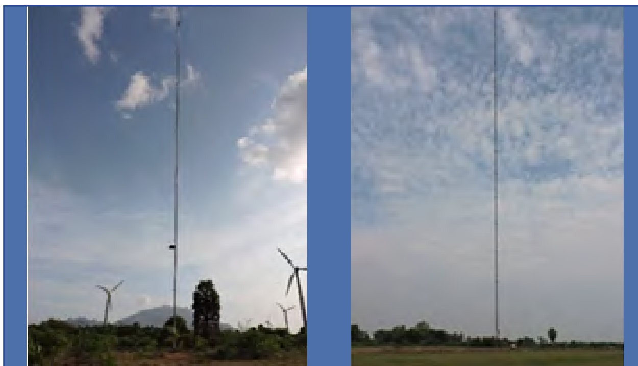
50m tubular mast at Perungudi
