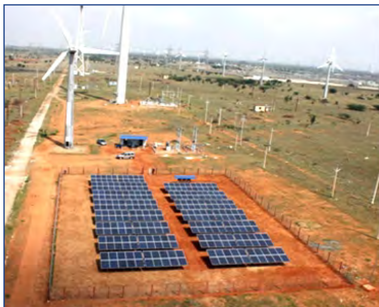
Grid Integration of 75 kWp Solar with 200 kW WEG
