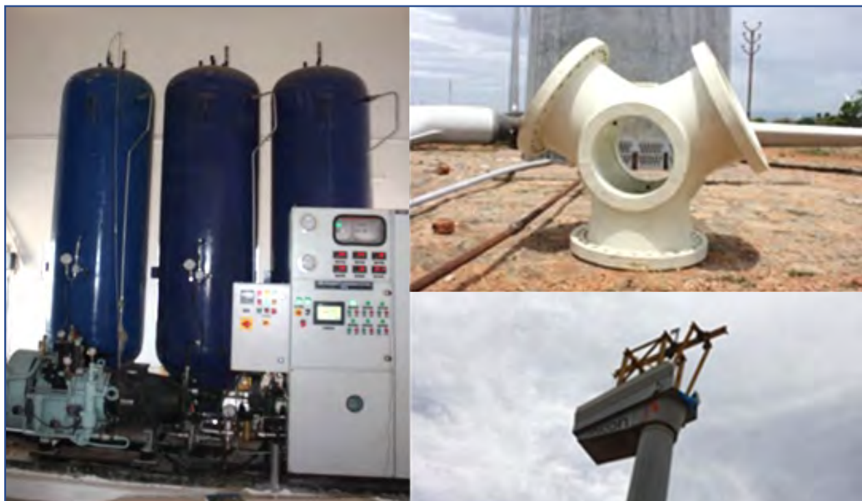
Erection of Cylinders, Compressor in the Control Room
