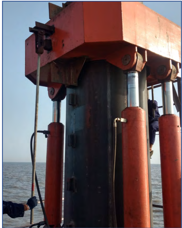
Hydraulic Pile driving mechanism
