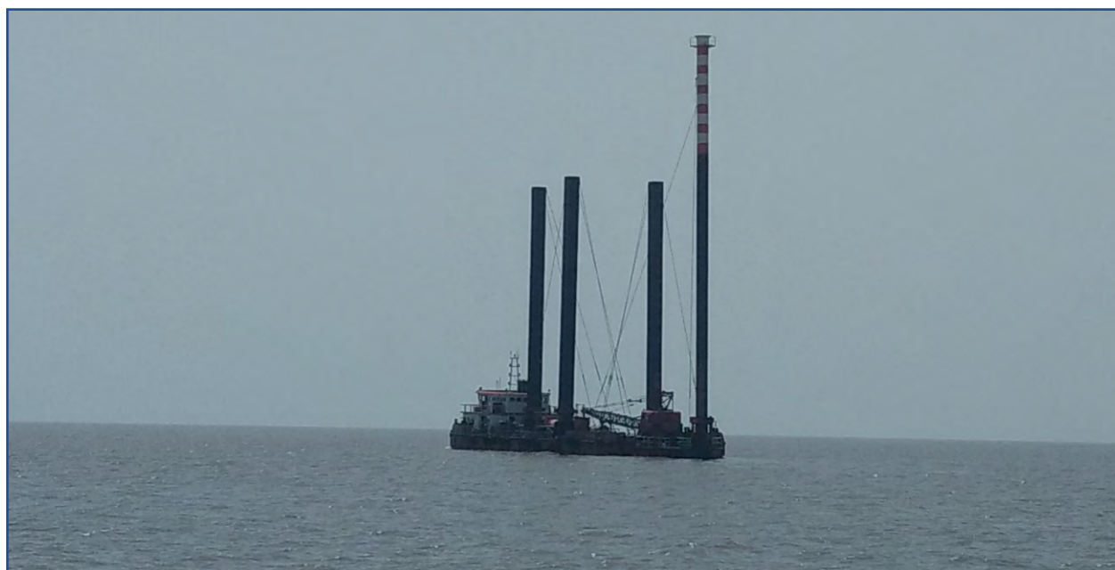
Jack up Barge Holding Structure
