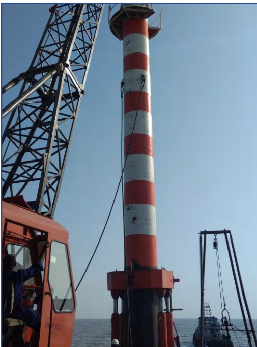
Hammering Monopile for Stability
