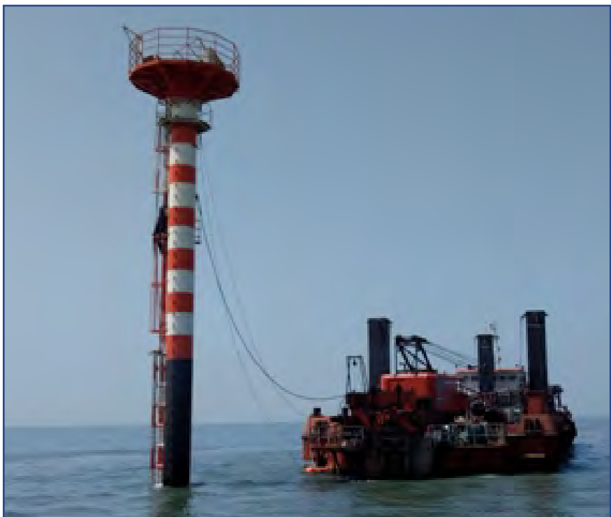
Completed Monopile and Platform
