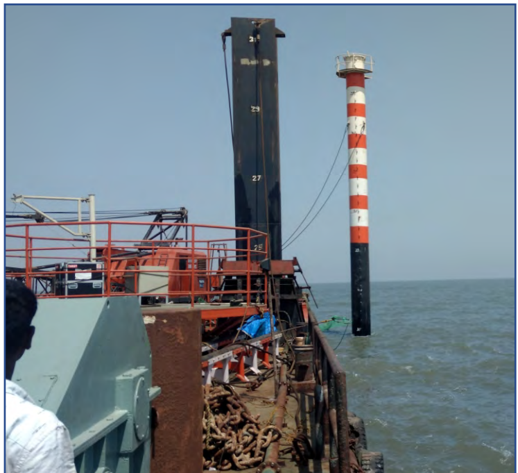
Completion of Monopile Installation
