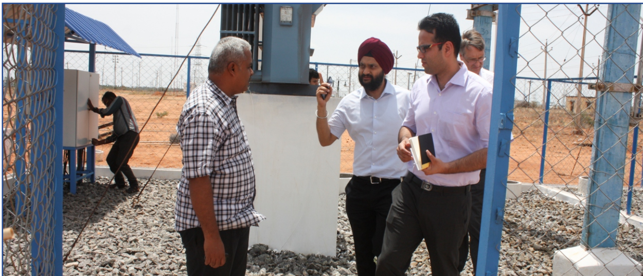
Visit of ICF, Fraunhofer to WTRS, Kayathar for VPP Project
