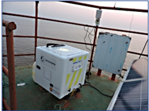
LiDAR at Offshore Platform
