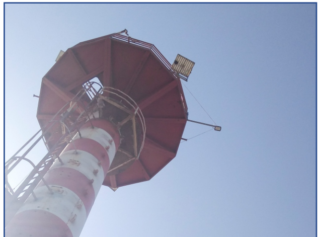
LiDAR substructure after installation of RADAR level sensor
