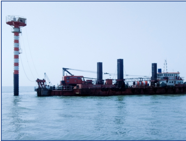
Monopile platform at Gulf of Khambhat
