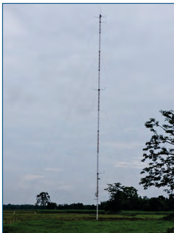
50m Mast Photograph of Bhurbanda, Assam
