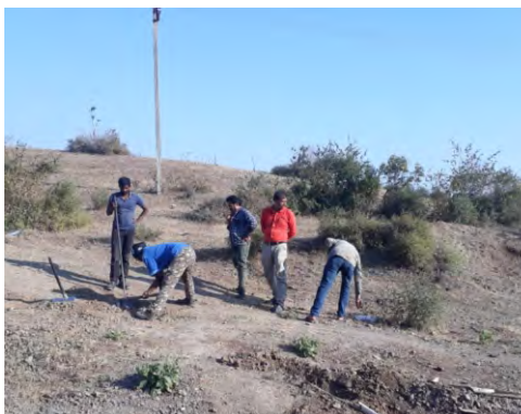
Atria RD113 control room to met mast cable laying – Power Curve Measurements of Inox 2000 kW wind turbine of M/s. Atria Wind Power (Savarkundla) Pvt. Ltd.
