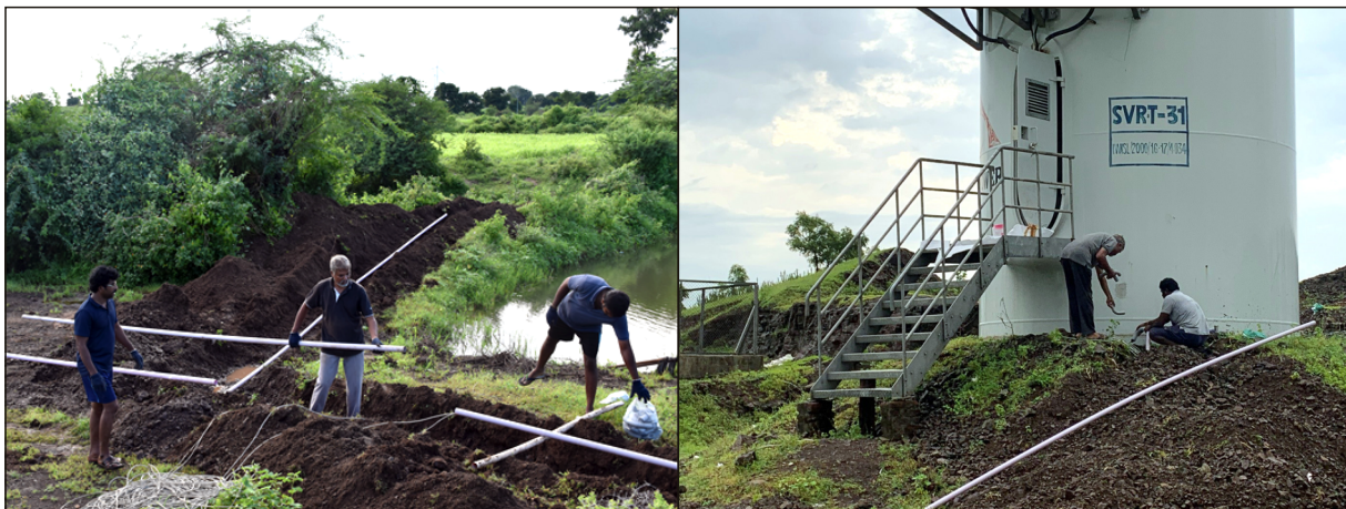
Cable Laying Work for Power Curve Measurement (PCM) for Model - INOX DF/2000/113, 2000 kW, a wind turbine from M/s. Inox Wind Ltd at Savarkundla, Amreli District Gujarat
