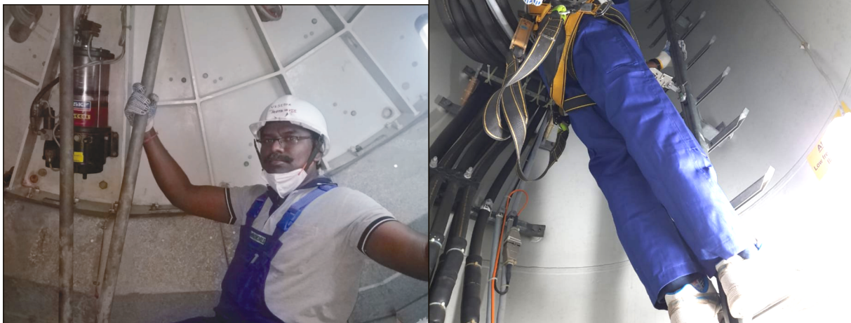
Conducted Onsite Inspection in connection with LTE Assessment
