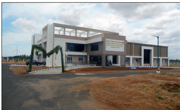
Renewable energy Demo lab building
