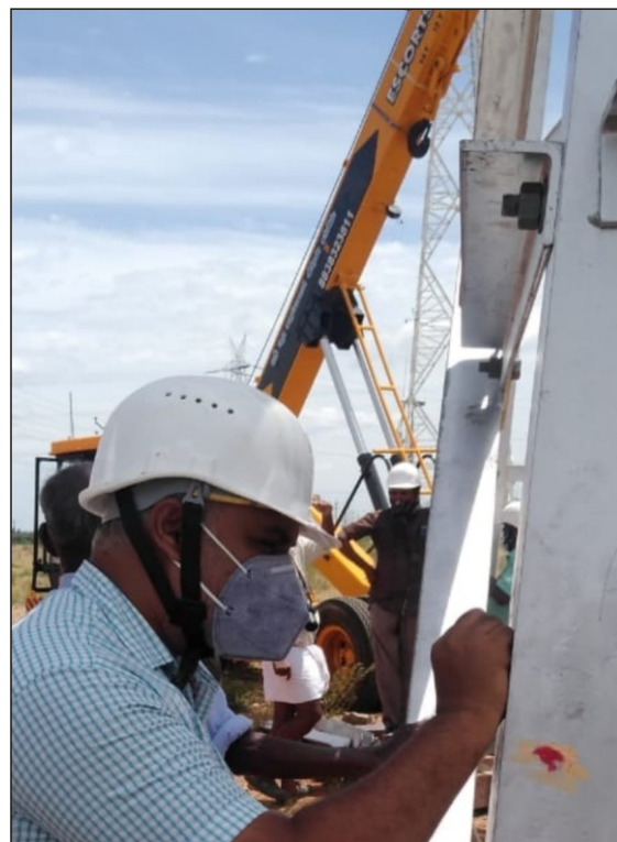
Strain Gauging work at tower legs
