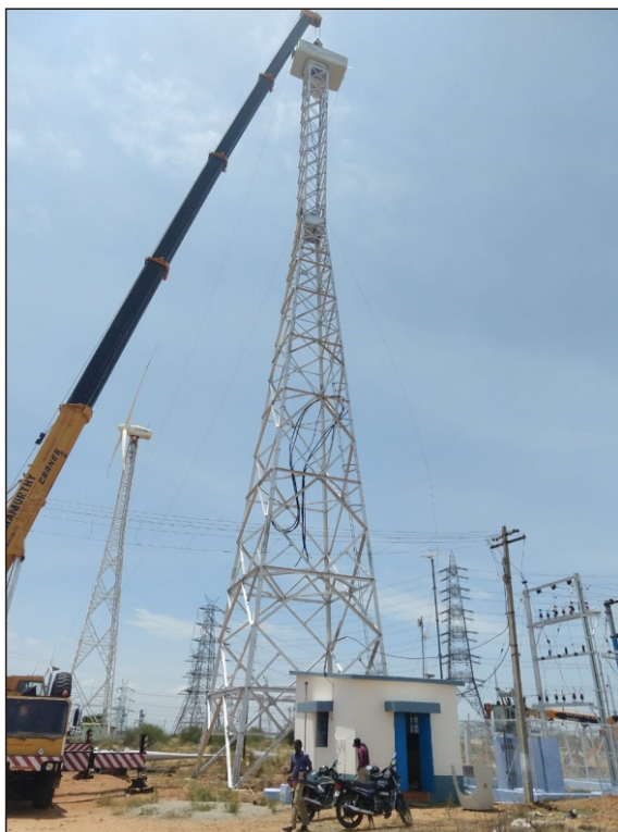
DST wind turbine instrumentation work
