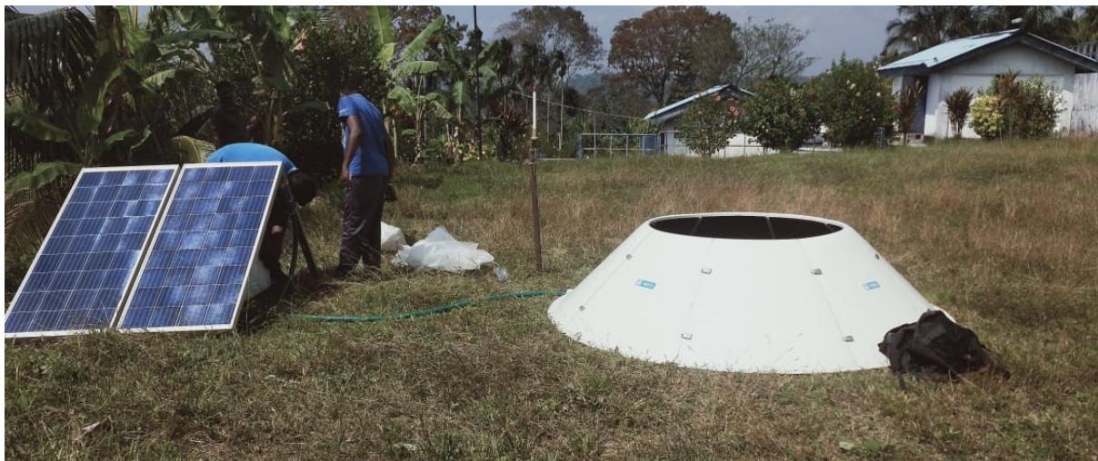
Installation of SoDAR at Guptapara site, A&N Islands
