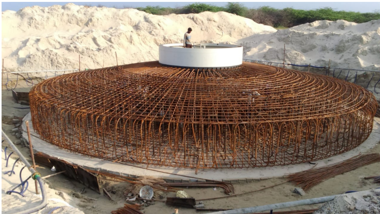
Foundation work progress at VOC Port Trust
