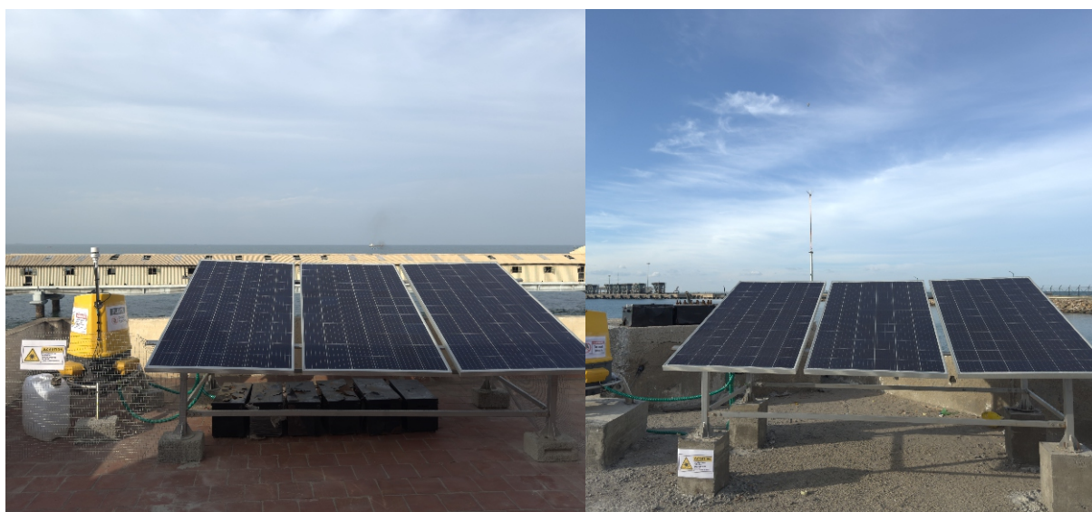
Lidar Installed at VOC Port, Gulf of Mannar, Off Tamil Nadu coast
