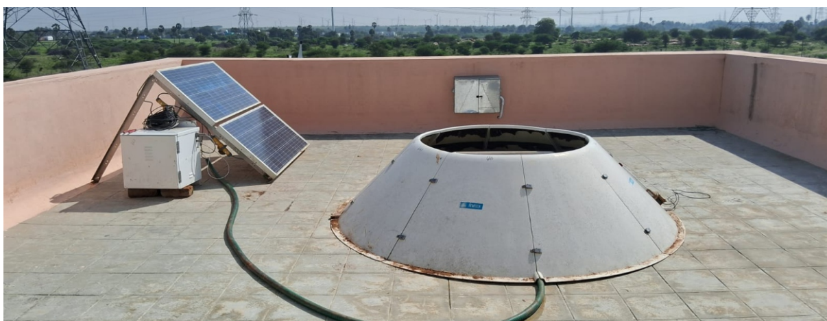
SoDAR system located at Kayathar
