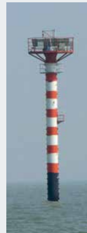
FIGURE 15-2: OFFSHORE LIDAR PLATFORM
