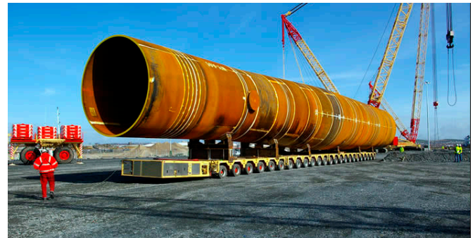
Figure 41 - Monopile onshore transport using SPMTs
