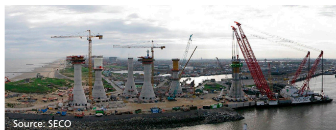
Figure 45 - Construction of GBS on the quay (Thornton Bank)
