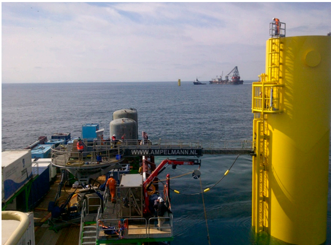
Figure 75 - Grouting spread on the aft of an offshore supply vessel - Borkum West II
