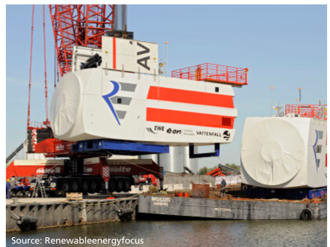
Figure 39 - Crawler crane nacelle load-out
