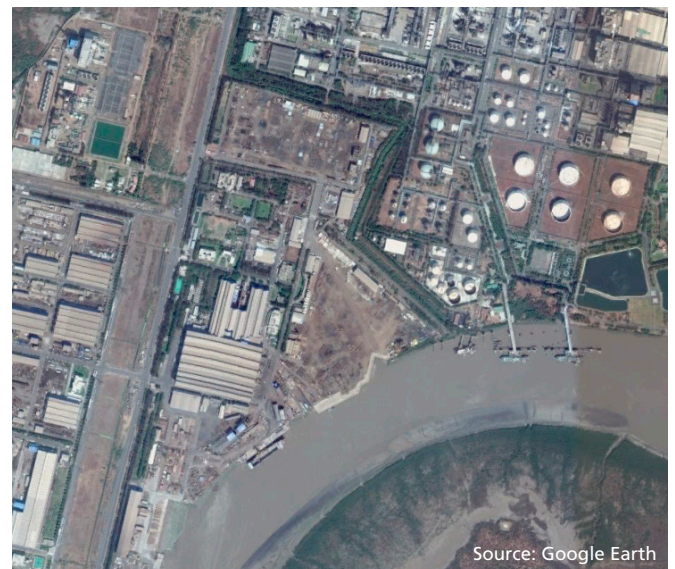
Figure 109 - Larsen & Toubro port and fabrication facility Hazira
