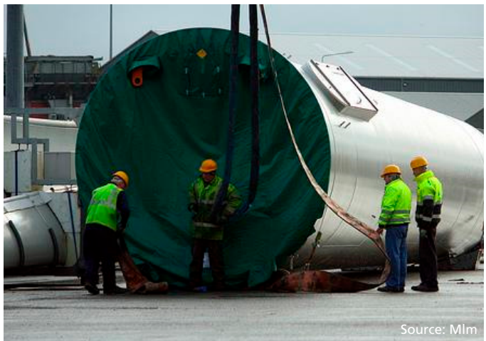
Figure 34 - Tower section storage
