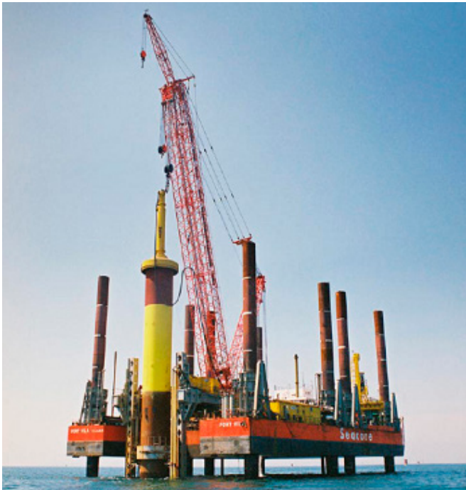
Figure 55 - Fugro Seacore's Excilibur towed jack-up installing a monopile
