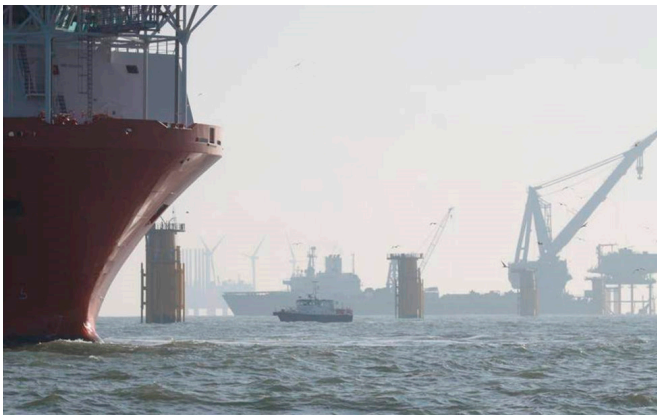
Figure 52 - Busy scene during construction of Thanet OWF
