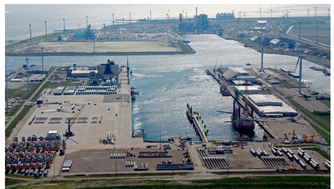
Figure 22 - Port of Eemshaven, WTG component marshalling
