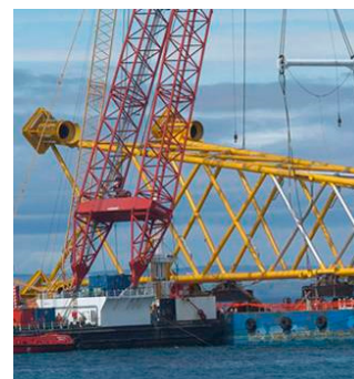
Figure 76 - Rambiz up-ending the leg-sheered jacket at Beatrice
