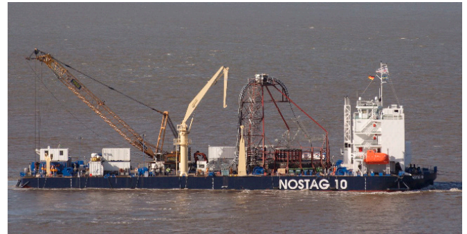
Figure 85 - Cable transportation and installation
