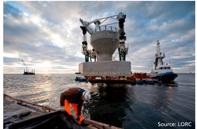
Figure 46 - GBS lift off construction barge using Eide 5 heavy-lift barge
