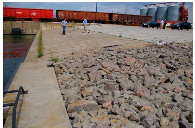
Figure 94 - Concrete ramp, used for RoRo load-outs
