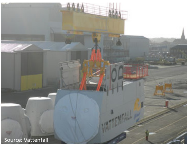
Figure 38 - Port crange nacelle load-out
