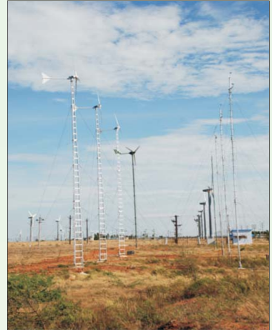
Array of SWT under test at WTRS
