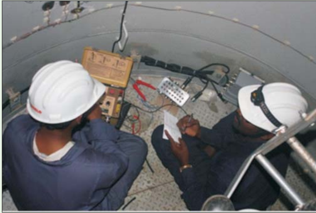
Tower top Strain Gauging
