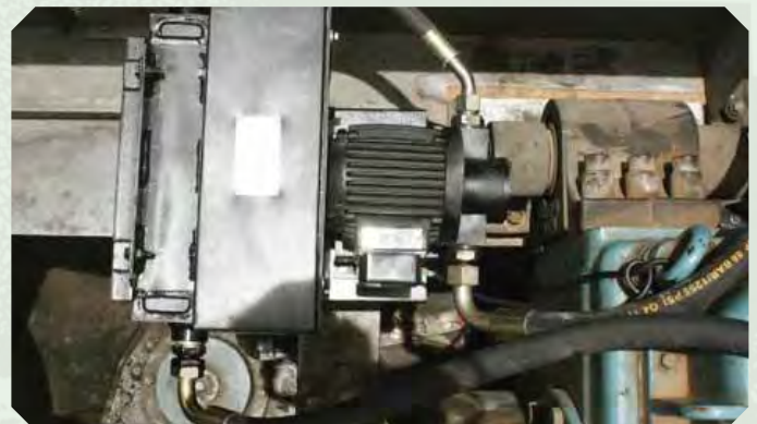
Installation of Gear Oil Cooling System at Nacelle
