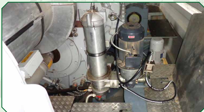
Wear Debris Sensor in the Gear Box Oil loop
