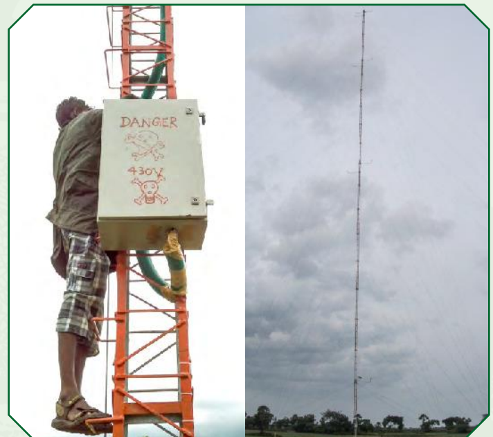
Commissioning of 100 m mast
