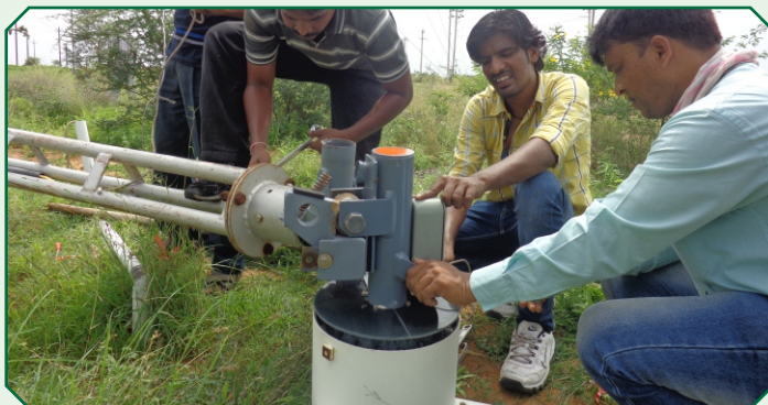
Dismantling process of the Model UE 42 at WTRS, Kayathar
