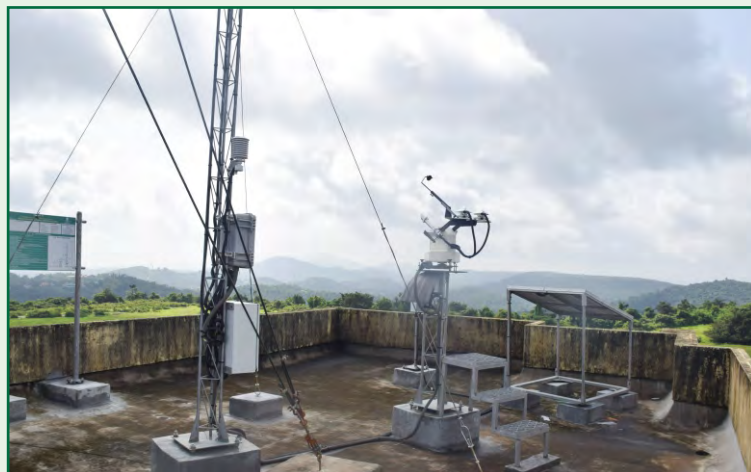
Panaji SRRA station
