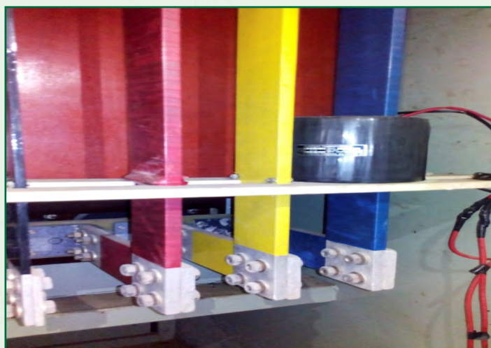
Electrical nodes identified for Energy Management System
