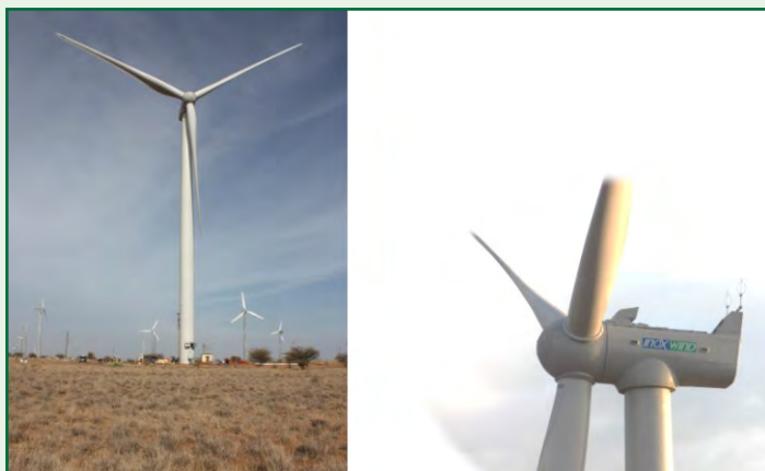
Erection of 2000 kW DFIG INOX WEG @ WTRS, Kayathar
