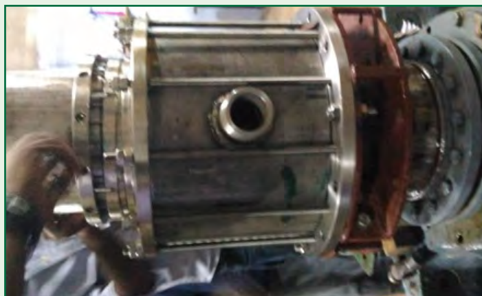
Installation of Micro Thruster Augmented at kW
