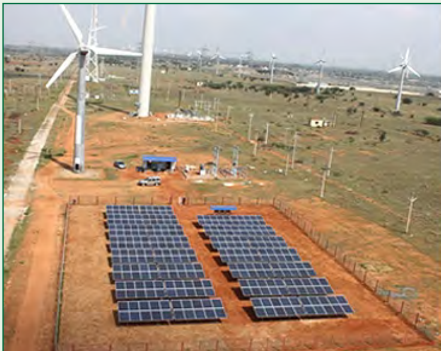
Grid Integration of 75 kWp Solar with 200 kW WEG
