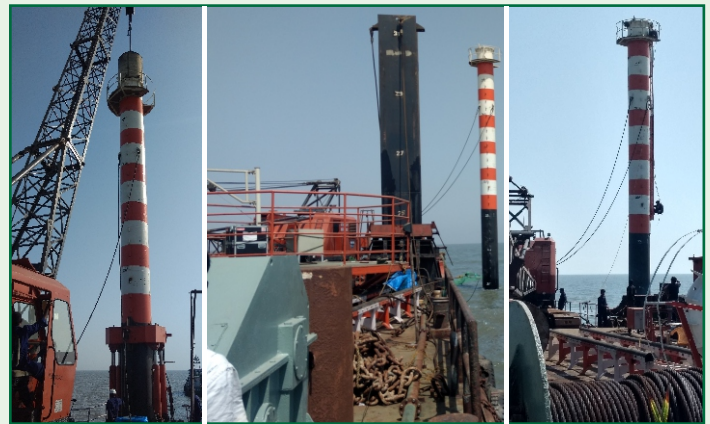
Hammering Monopile for Stability
