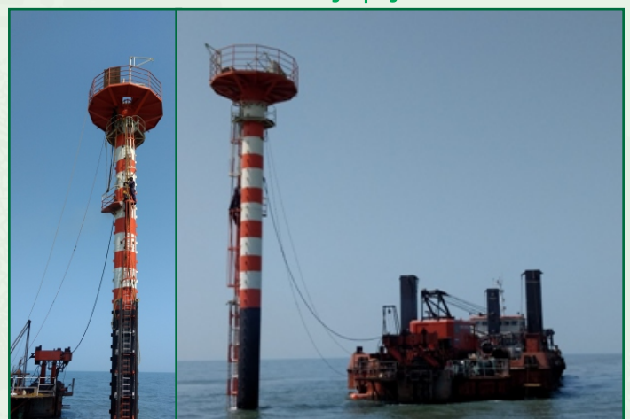
Fixing Boat Landing and Resting Platform
