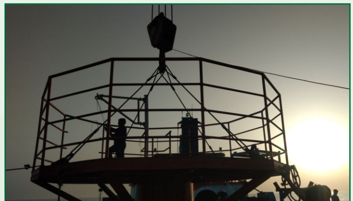
Platform Mounting in progress
