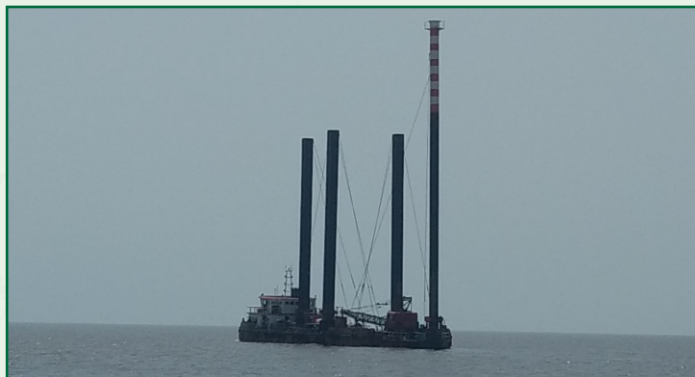
Jack up Barge Holding Structure
