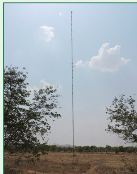
100m Wind Monitoring Station in Chattisgarh
