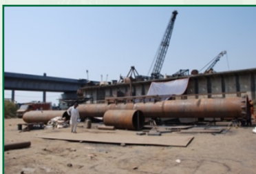
Figure 6 Fabrication of Sub-Structure
