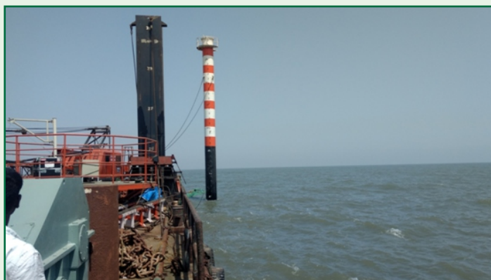
Figure 15 Monopile Released from Barge
