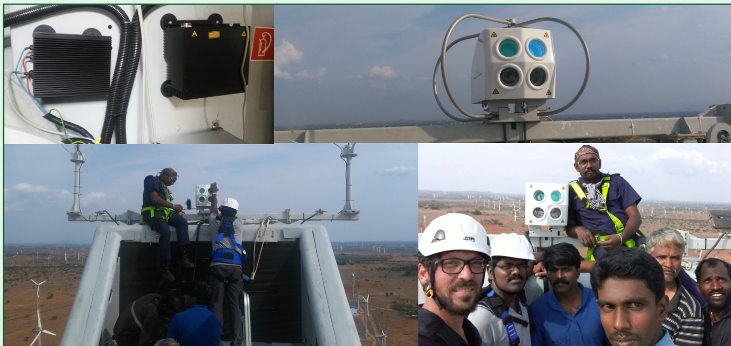
Installation & Commissioning of Nacelle based LIDAR installed on INOX R&D wind turbine by Mr. Sergio Martinez, Windar Photonics, Spain at Wind Turbine Test Station (WTTS), Kayathar
