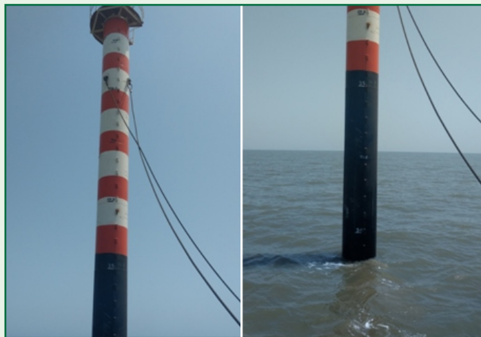
Figure 14 Installed Monopile
