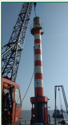
Figure 13 Hammering the Monopile
