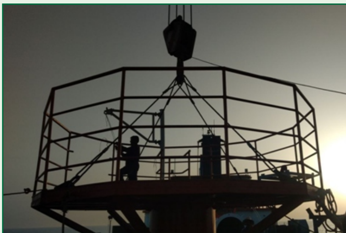
Figure 17 Lifting of Platform
