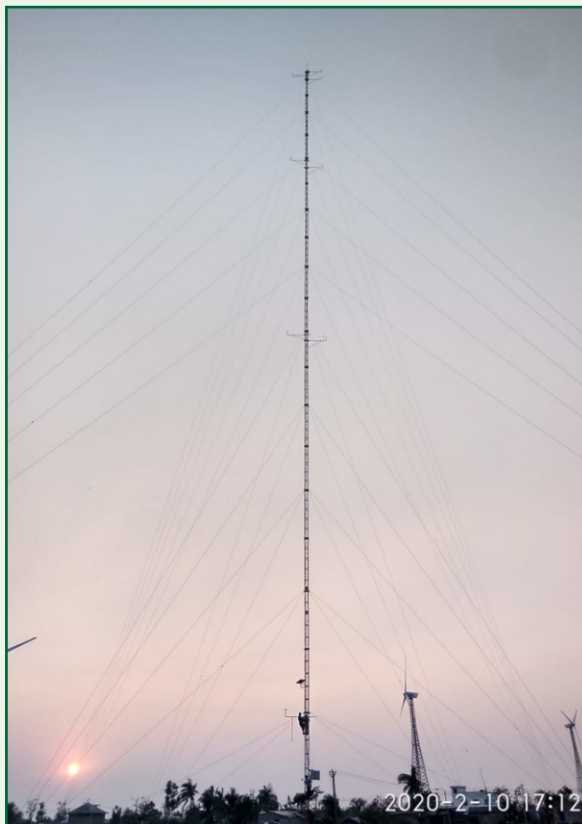
100 m Wind monitoring station installed at West Bengal
