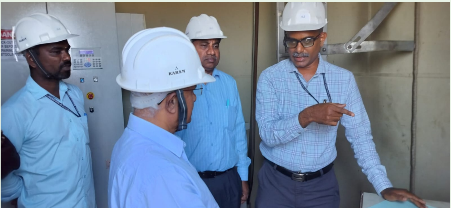
First Periodic Audit conducted by M/s. DNV Business Assurance India Private Limited at WTTS, Kayathar on 01.06.2026
