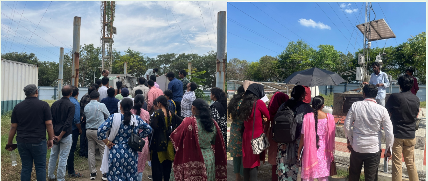
Glimpse of RE facility visit at NIWE
