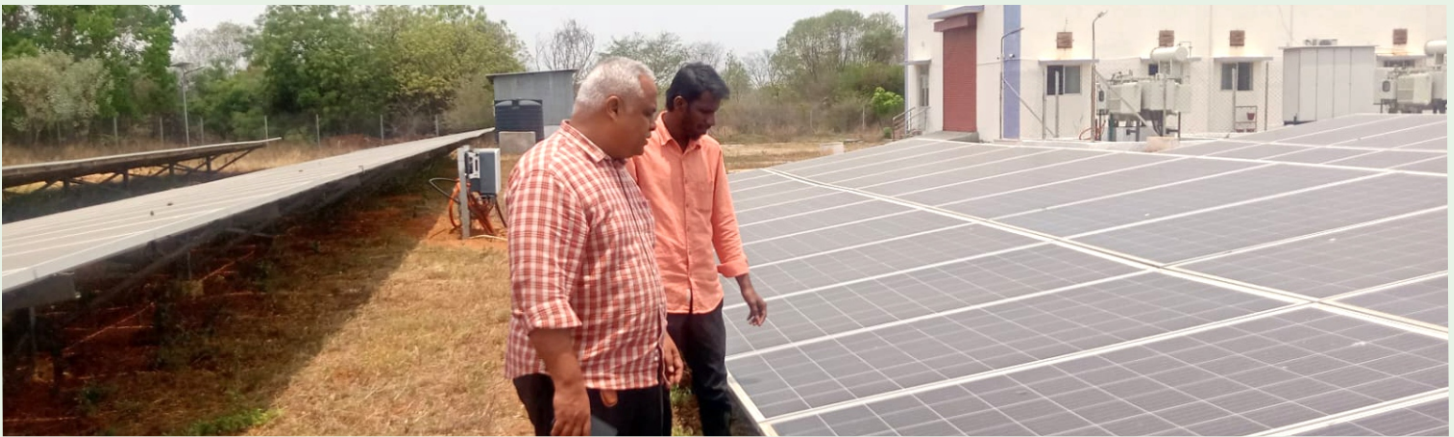
Joint Inspection carried out MKU Madurai on 29.04.2026
