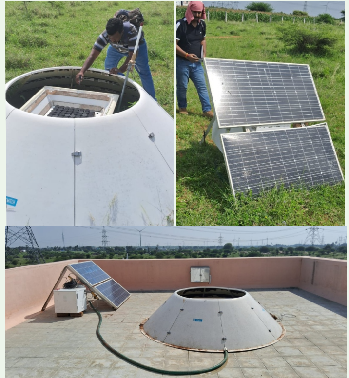
SoDAR rectification work at Kayathar
