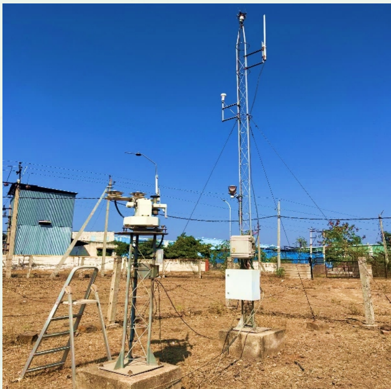
SRRA Station Installed in Karnataka
