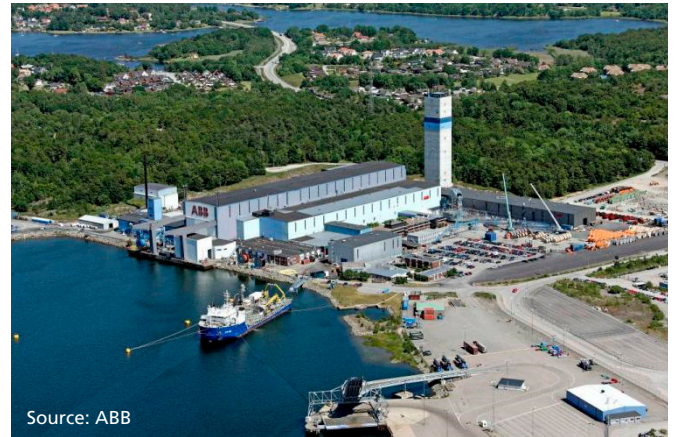
Figure 51 - ABB's high-voltage manufacturing facility in Sweden
