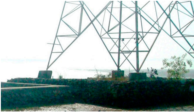
Figure 99 - Structure in the river showing heavy scour protection
