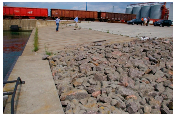
Figure 94 - Concrete ramp, used for RoRo load-outs
