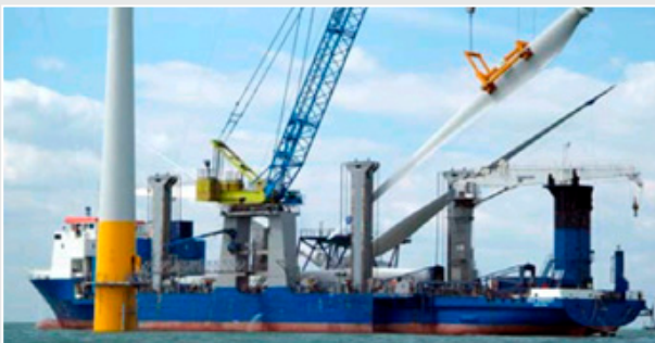
Leg-stabilised crane vessel
