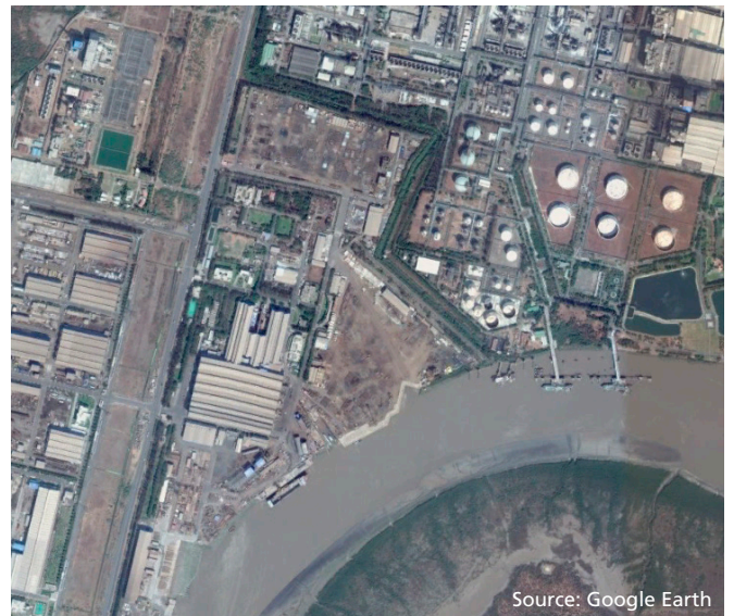
Figure 109 - Larsen & Toubro port and fabrication facility Hazira
