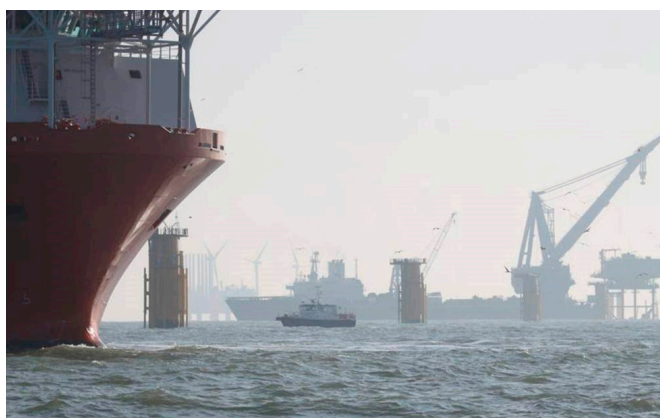
Figure 52 - Busy scene during construction of Thanet OWF
