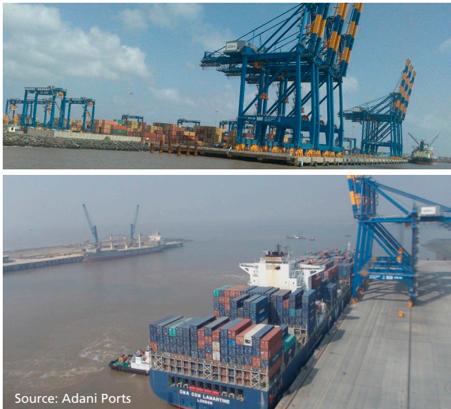
Figure 107 - Adani container berths with cranes
