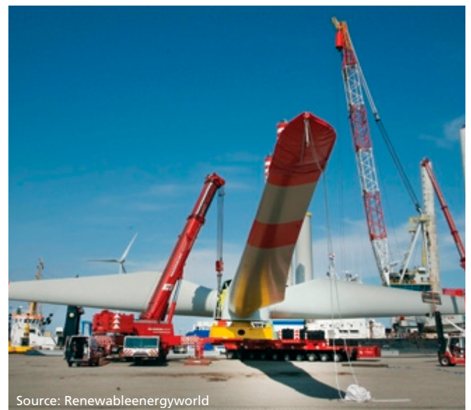
Figure 31 - Full rotor assembly in port
