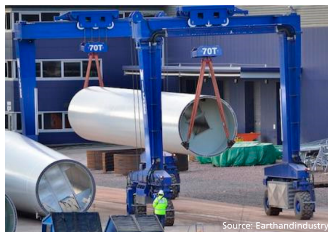
Figure 33 - Tower section transportation
