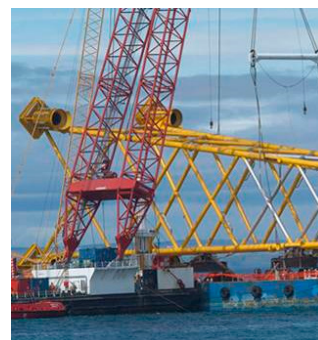
Figure 76 - Rambiz up-ending the leg-sheered jacket at Beatrice
