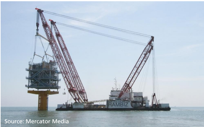
Figure 61 - Rambiz 3, 300 t SHLV installing a substation topside
