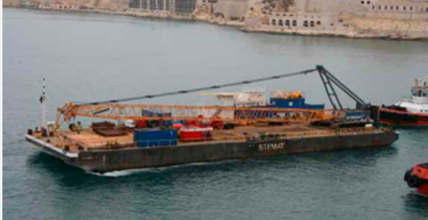
Towed 'dumb' barge with crane
