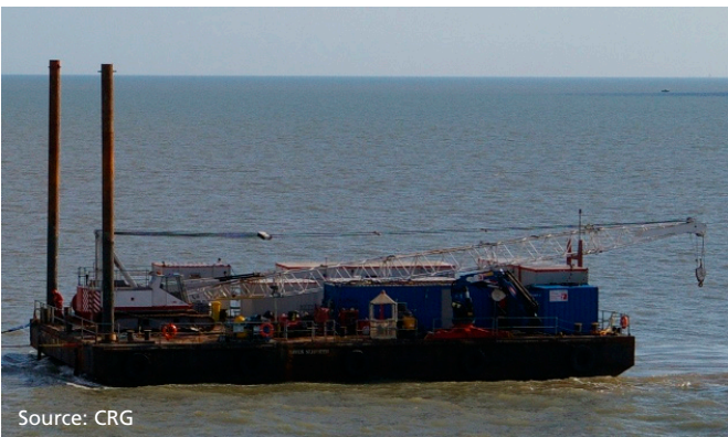
Figure 54 - Dumb barge with spud-legs, and crawler crane
