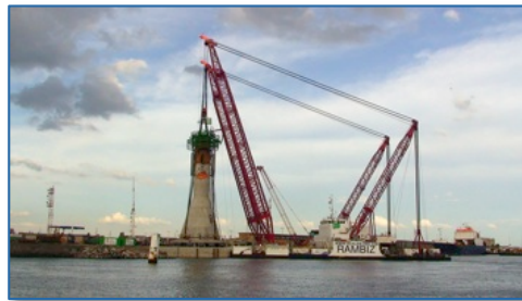
Lift GBF from quay wall
