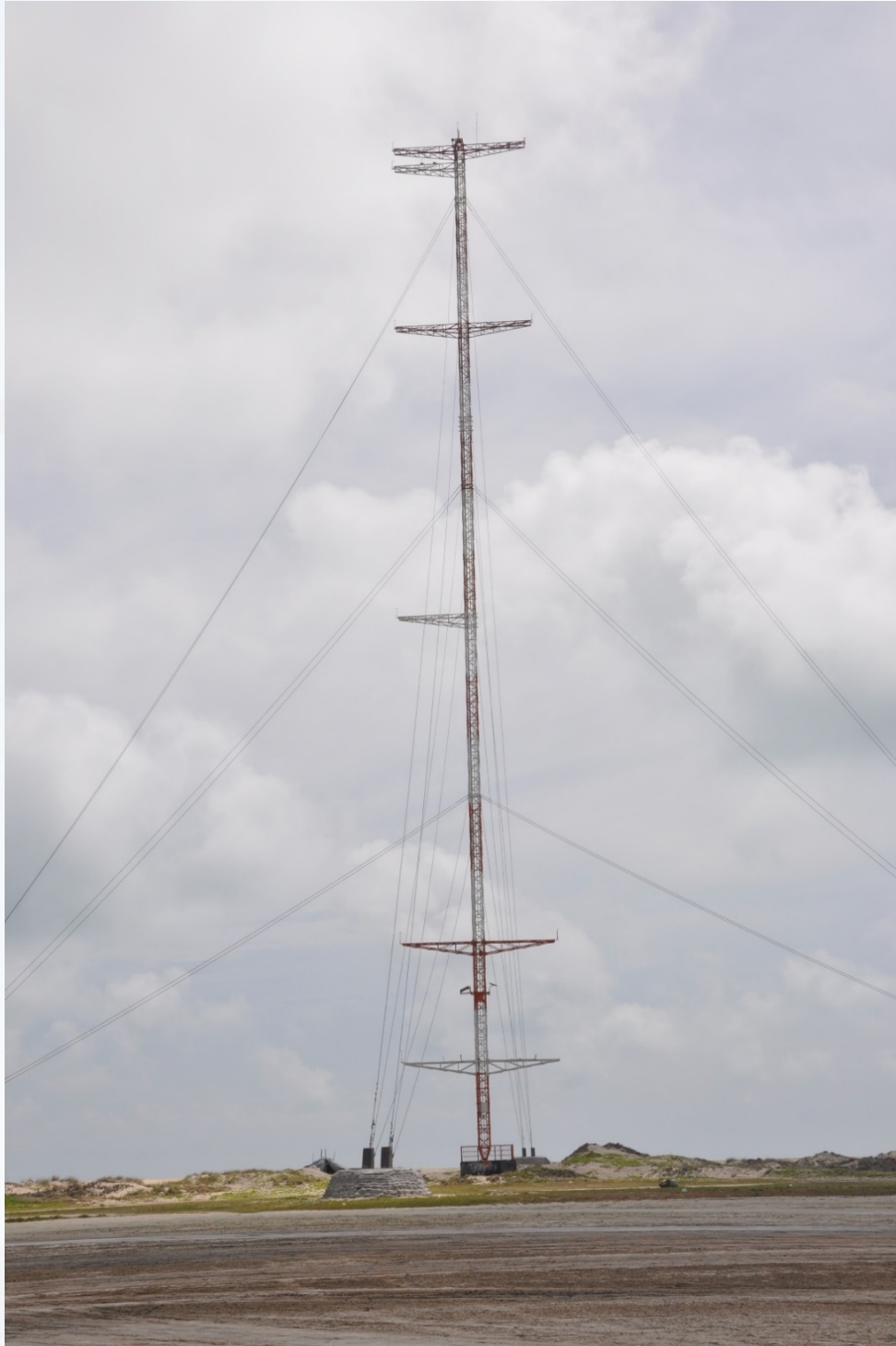
Figure 7: Image of Dhanushkodi 100m Mast
