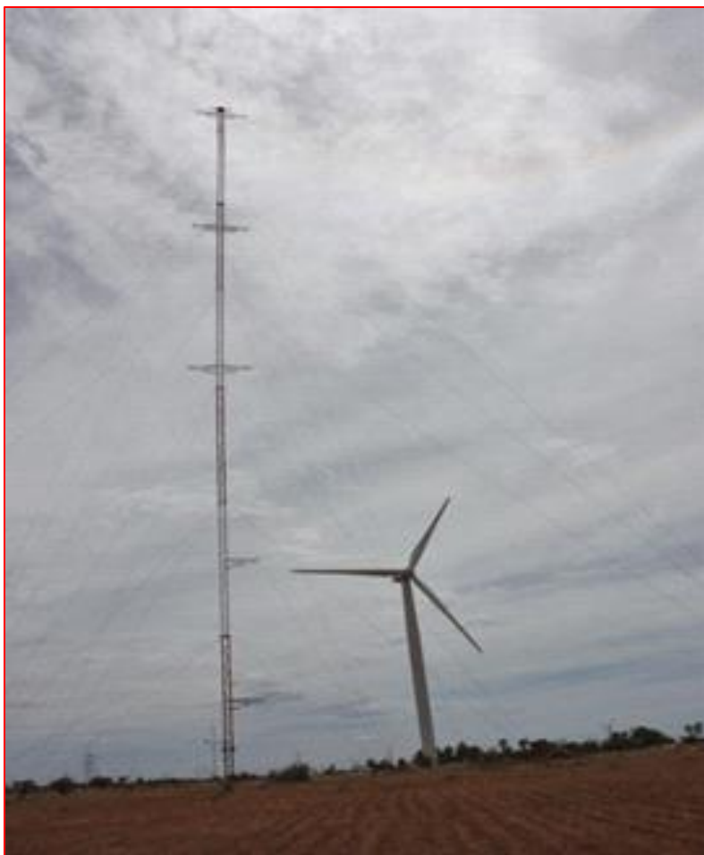
Figure 1: LiDAR set up
