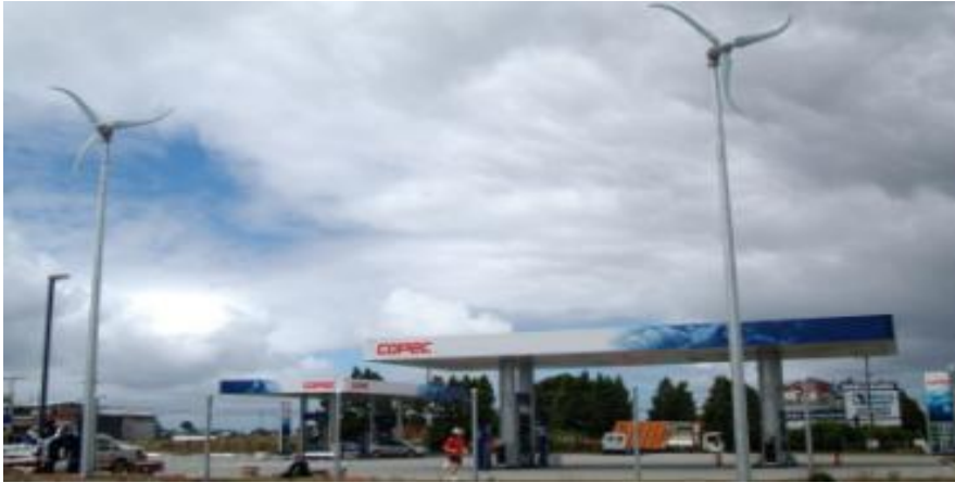
Supplemental “power plants” in infrastructure-strained urban areas
